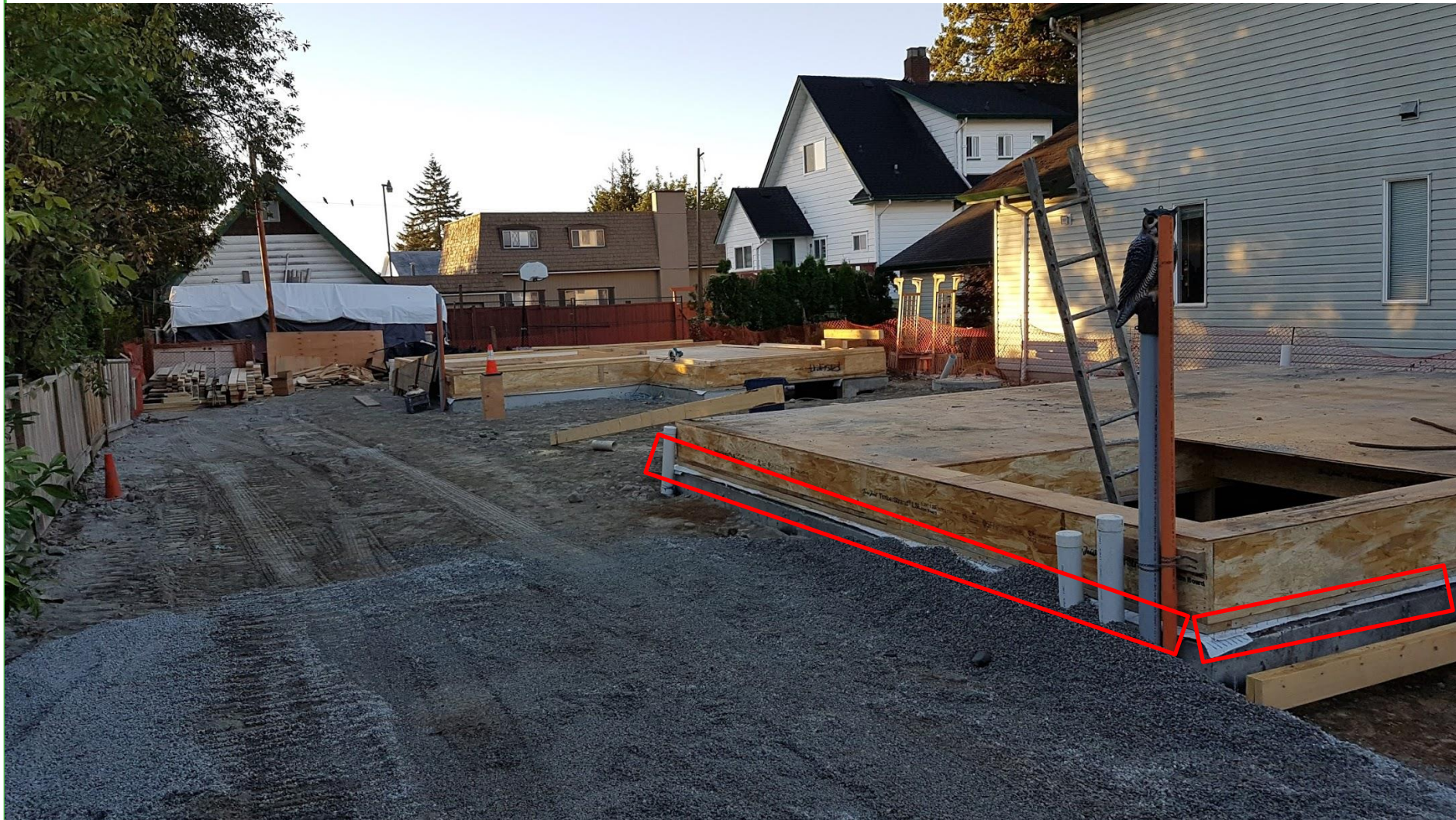
Thru-wall flashing and foundation
