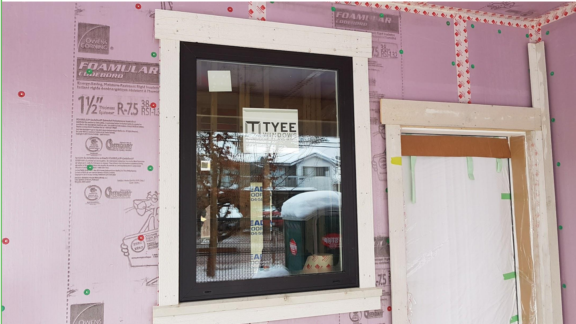
Face nailing of all exterior cladding components.
