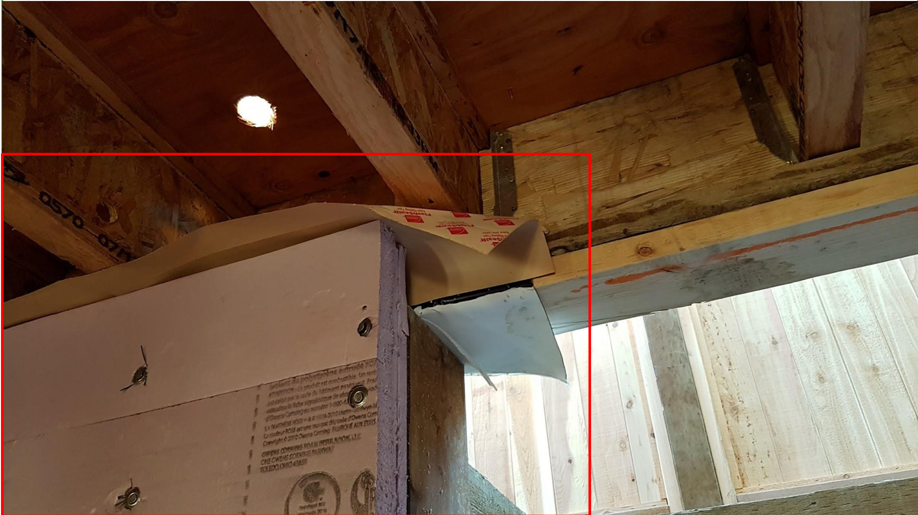
Transition of exterior air barrier to inside.
