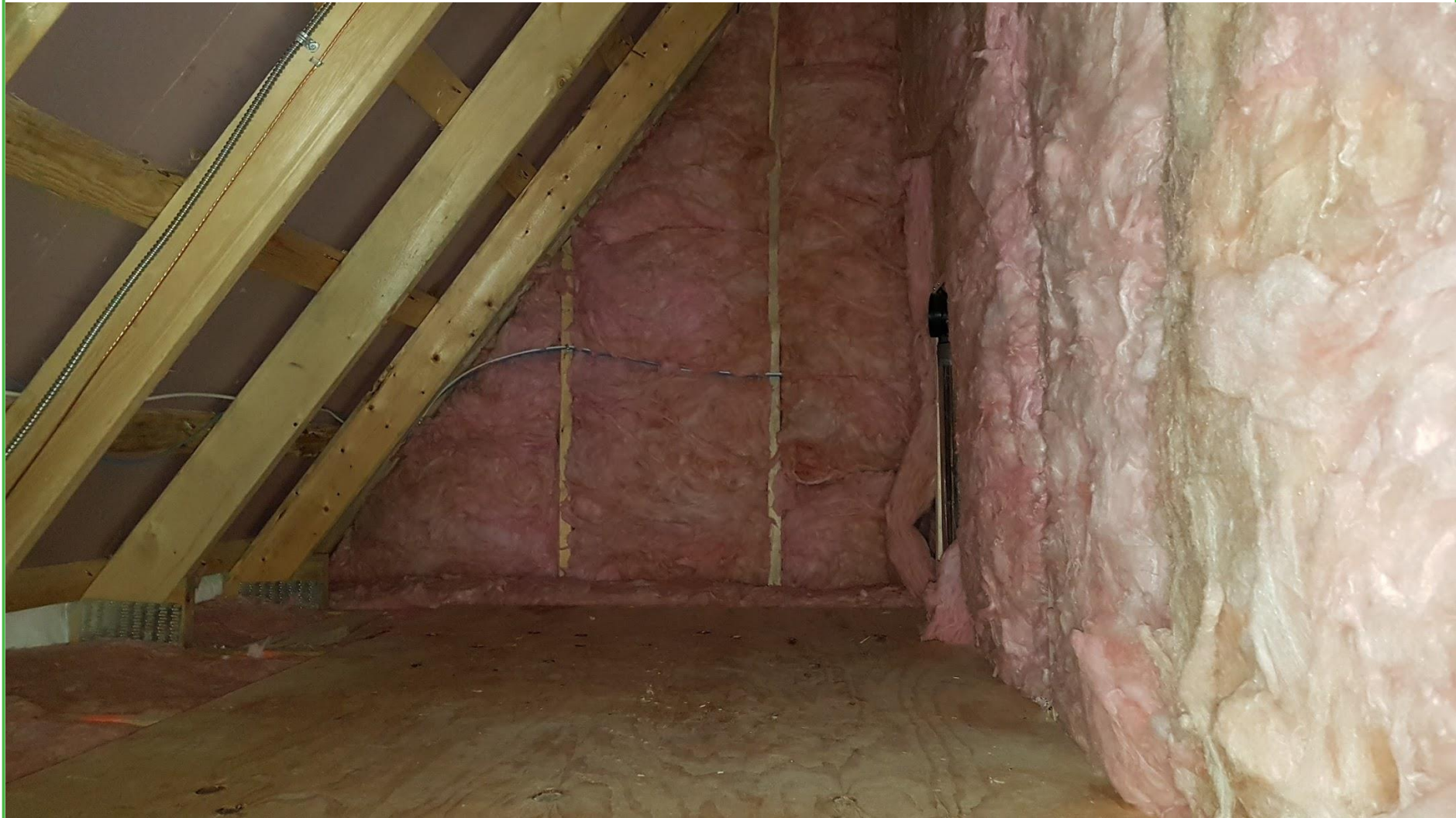
Inside the conditioned attic space, showing roof and exterior walls insulation.
