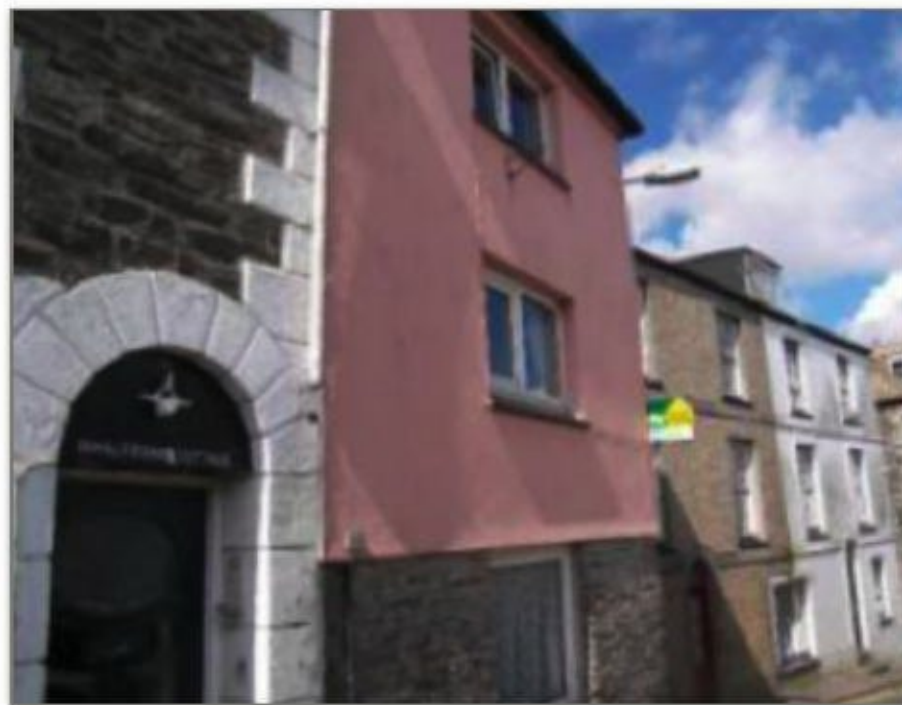
Picture 8 Old front wall elevation aspect while painted in pink
