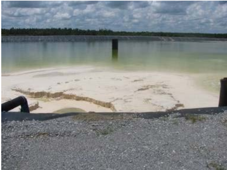
Photo 177: Surface of Gypsum Storage Pond looking west.
