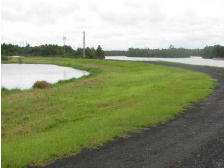
Photo 69: Crest of Ash Pond near east corner of pond looking north.
