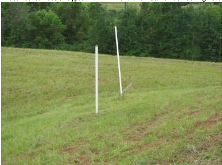
Photo 107: Piezometers on south exterior slope of Gypsum Pond looking south.
