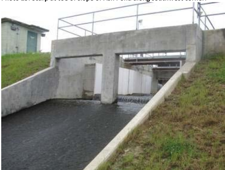
Photo 31: Spillway and discharge channel of outfall structure.
