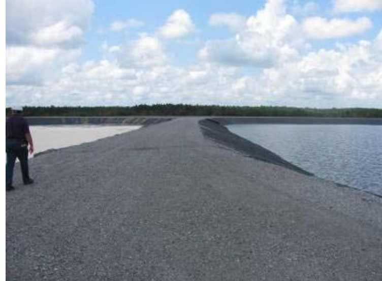
Photo 164: Intermediate embankment between Gypsum Pond and Process Sedimentation Pond looking northwest.
