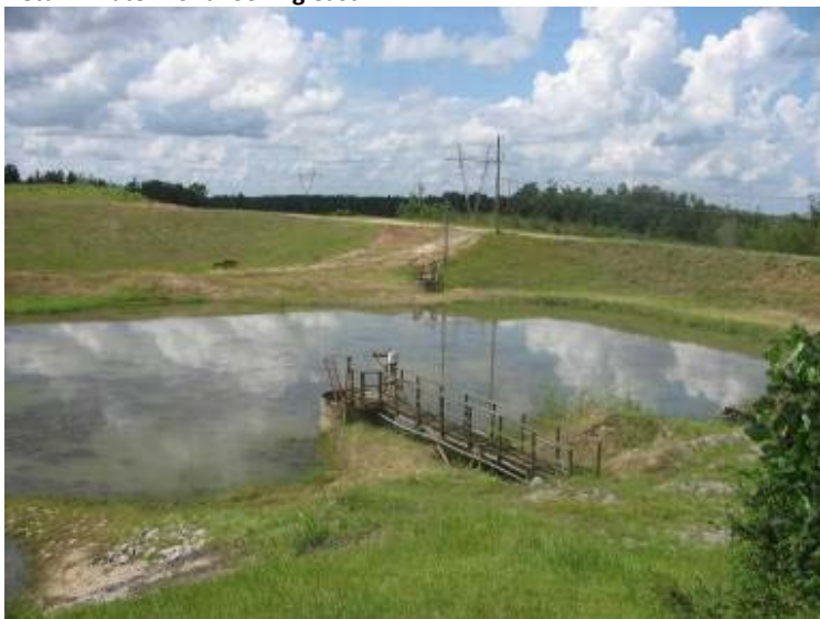
Photo 195: General view of fly Ash Landfill stormwater pond area looking northwest.
