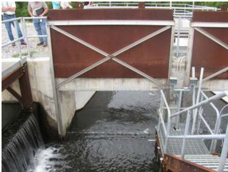
Photo 39: Spillway structure looking downstream.
