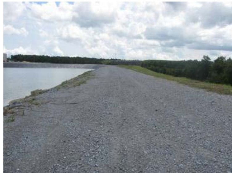
Photo 172: Crest of west embankment of Gypsum Storage Pond looking south.
