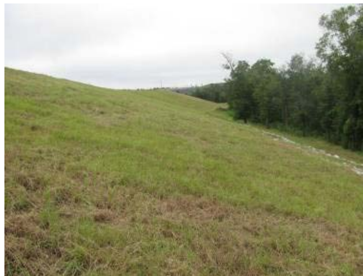
Photo 126: Exterior slope along west side of Gypsum O Pond looking south.
