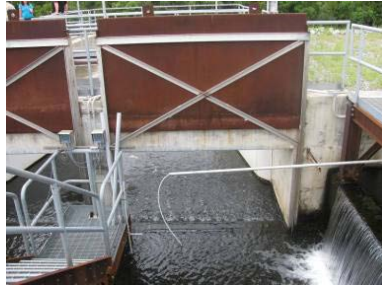
Photo 38: Spillway structure looking downstream.
