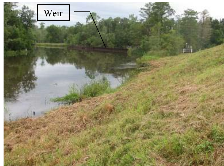
Photo 28: View of sheet pile discharge weir looking south.
