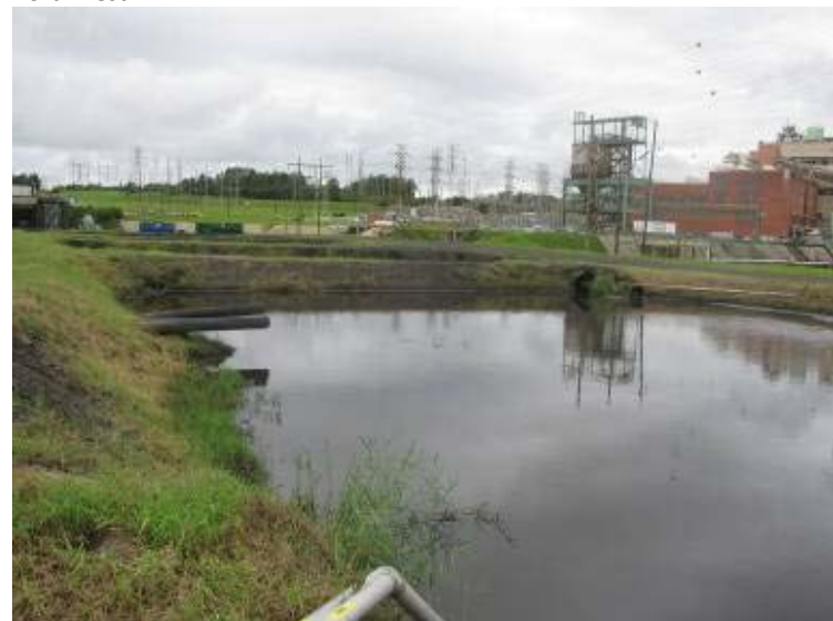
Photo 80: Surface and southeast interior slope of Decant/Settling Pond #5.
