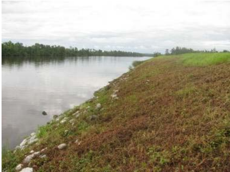
Photo 9: View of exterior slope of Ash Pond north embankment looking east.
