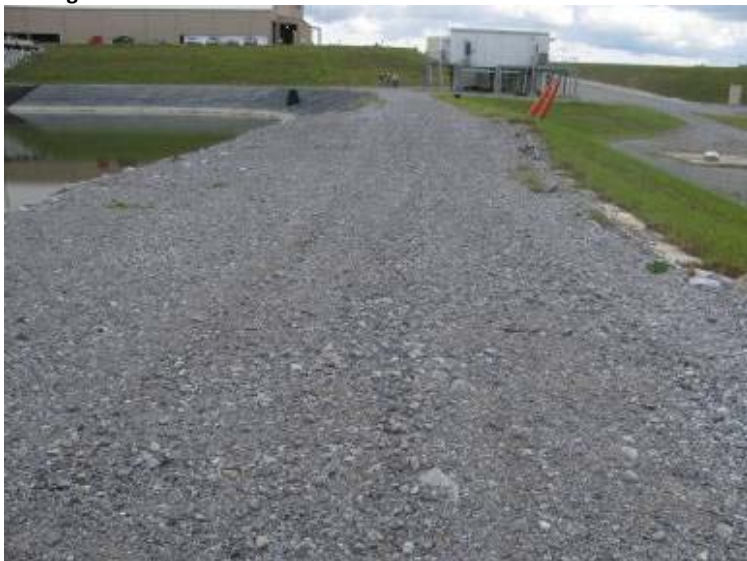
Photo 187: Crest and emergency spillway along west embankment of Process Return Water Pond looking south.
