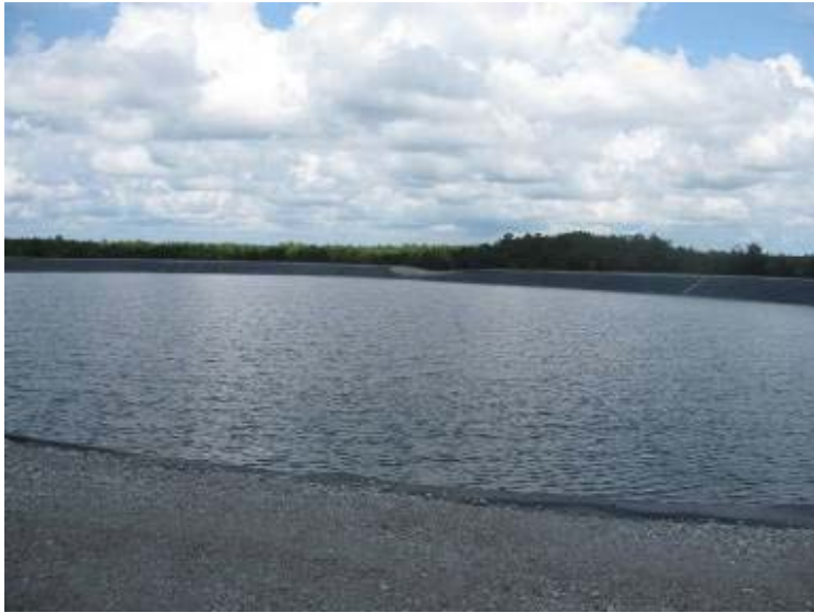
Photo 165: Surface of Process Sedimentation Pond looking north.
