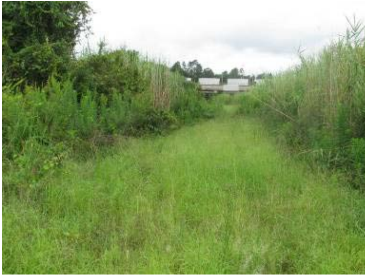
Photo 85: Crest of Ash Pond along northwest side. Note dense vegetation.
