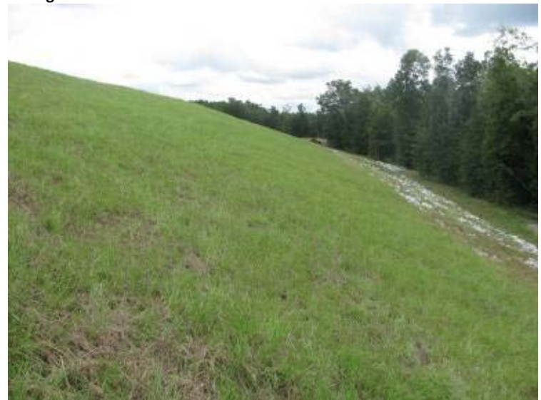
Photo 160: Exterior slope of south embankment of Process Sedimentation Pond looking east.
