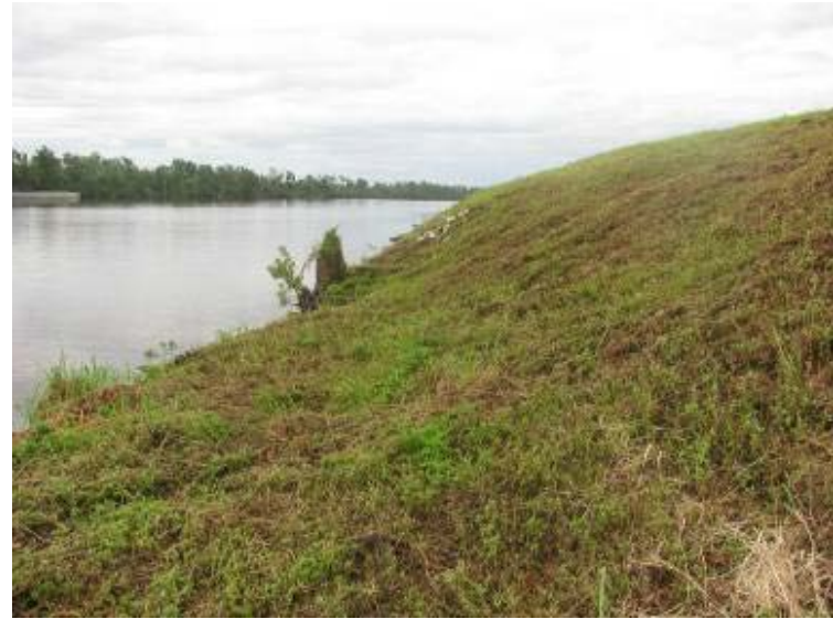
Photo 6: View of exterior slope of Ash Pond north embankment looking east.
