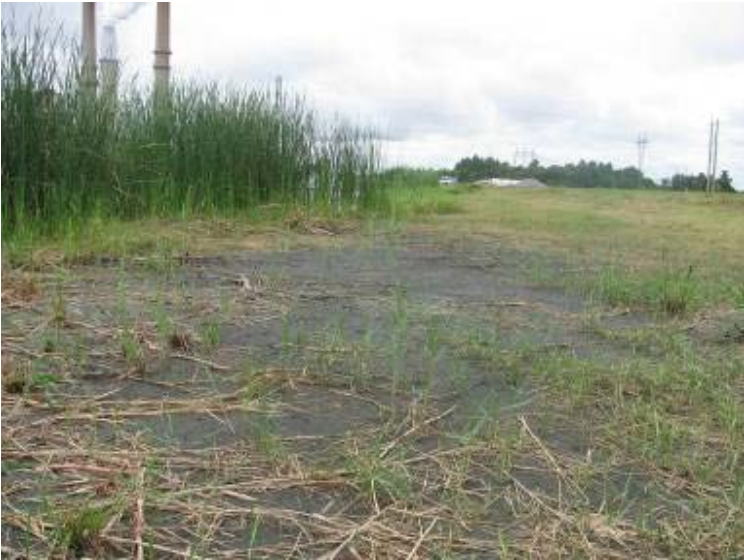
Photo 73: Ash delta located along interior slope of northeast embankment of Ash Pond looking northwest.
