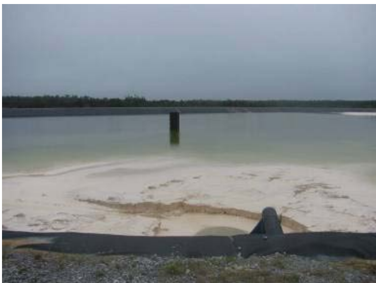
Photo 103: View of surface of Gypsum Pond looking west. Note discharge pipe & deposition of gypsum in foreground and Decant Riser in center of photo.
