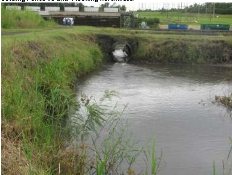
Photo 95: Interior slope and surface of Decant/Settling Pond #4 looking southwest.
