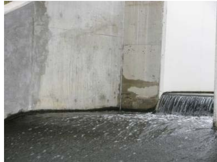
Photo 34: Ash Pond spillway looking north.
