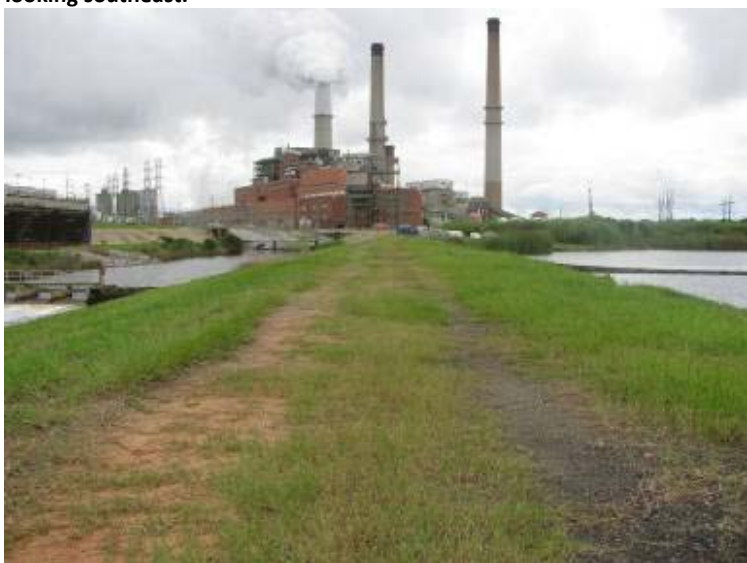
Photo 55: Crest of Ash Pond along southwest embankment looking northwest.
