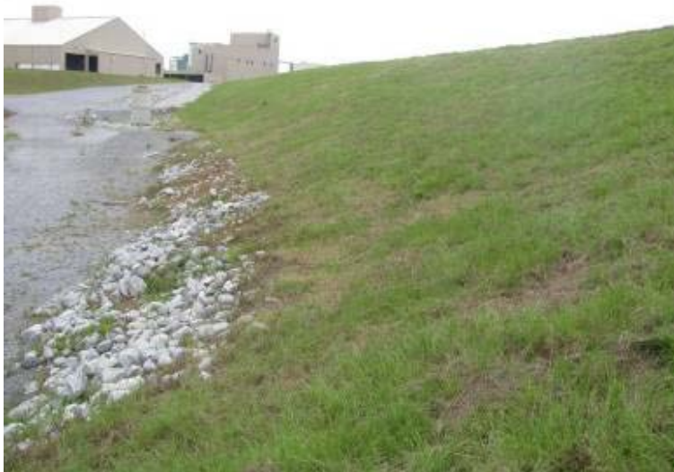
Photo 159: Exterior slope of east embankment of Gypsum Storage Pond looking southeast.
