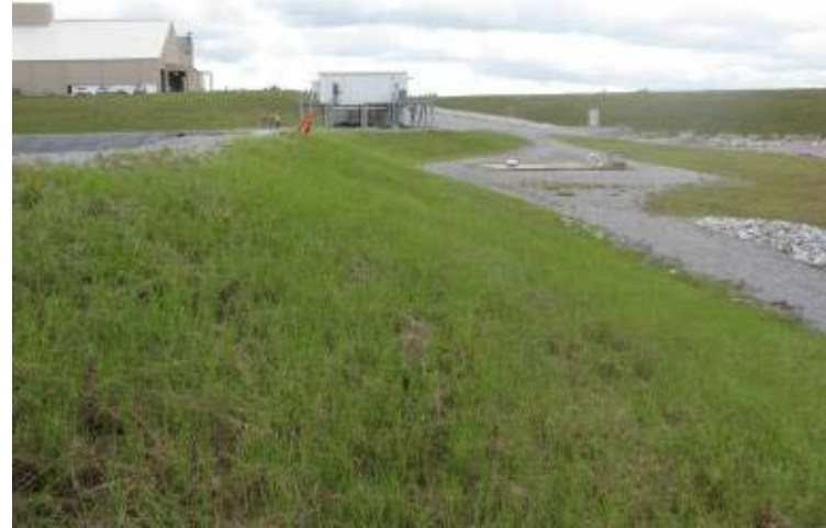
Photo 186: West exterior slope of Process Return Water Pond looking south.
