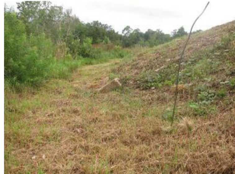
Photo 24: Exterior slope of Ash Pond along southeast embankment looking southwest.
