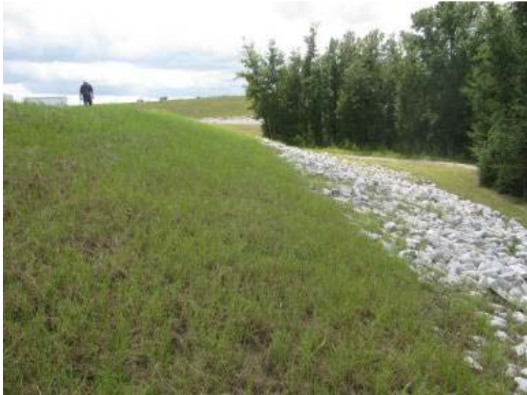
Photo 185: Northwest exterior slope of Process Return Water Pond looking southwest.
