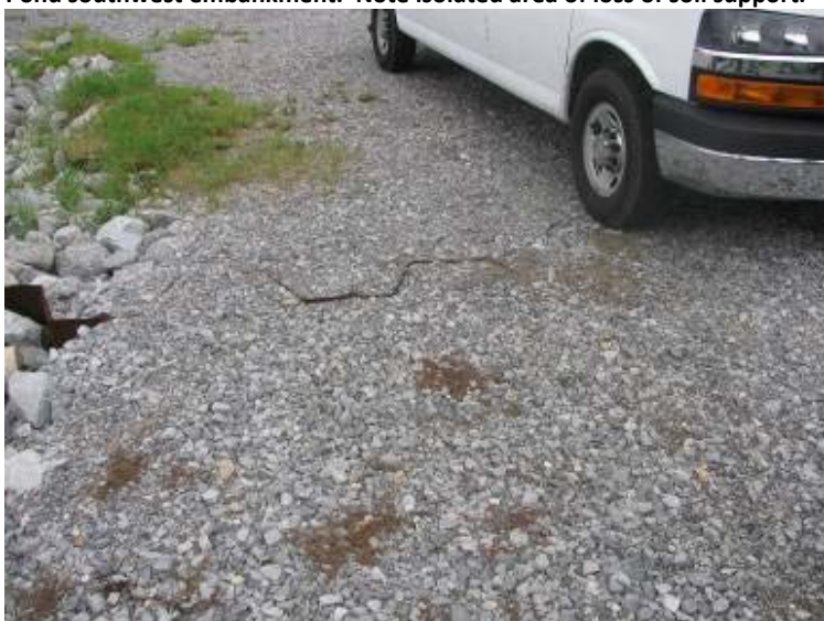
Photo 63: Portion of abandoned sheet pile cofferdam left in place on south side of spillway used to construct spillway.
