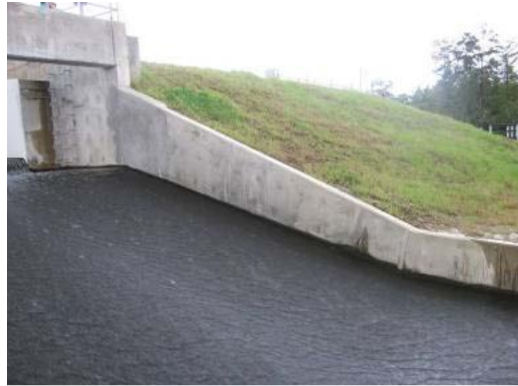
Photo 42: Downstream side of Ash Pond spillway.
