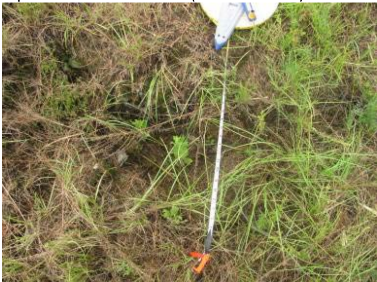
Photo 135: Rill located on north exterior slope of Process Sedimentation Pond (typical of six).
