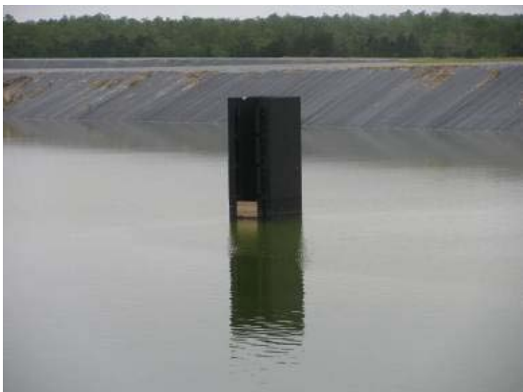
Photo 105: Surface of Gypsum Pond and Decant Riser looking north.
