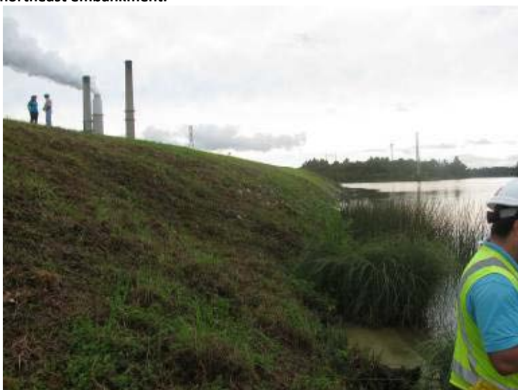
Photo 19: Exterior slope of Ash Pond along northeast embankment showing scarp with sand fan at toe of slope looking northwest.
