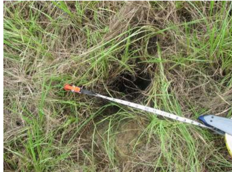
Photo 154: Animal burrow located at toe of slope east exterior slope of Gypsum Storage Pond.
