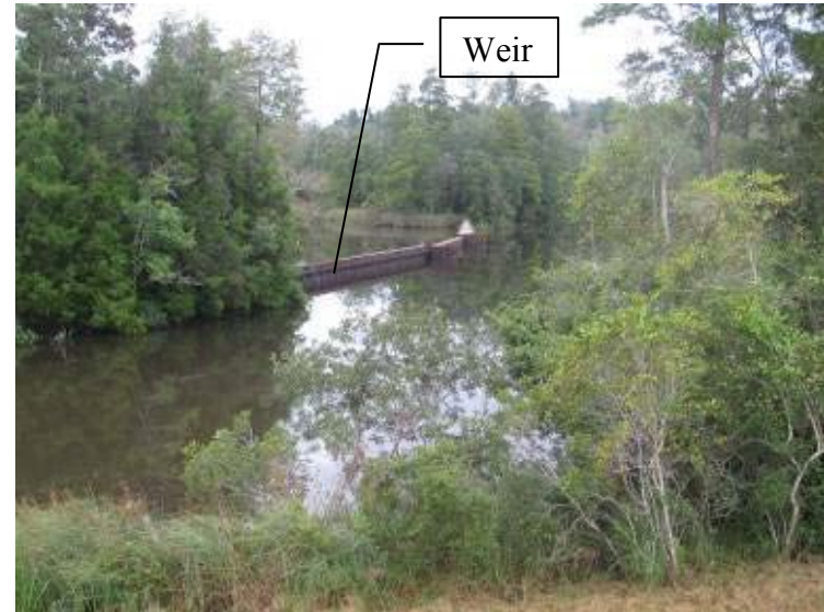
Photo 30: Downstream view of discharge weir for outfall looking southeast.
