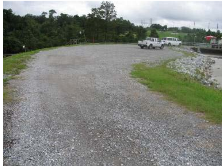
Photo 66: Crest of Ash Pond near south corner of pond looking west.
