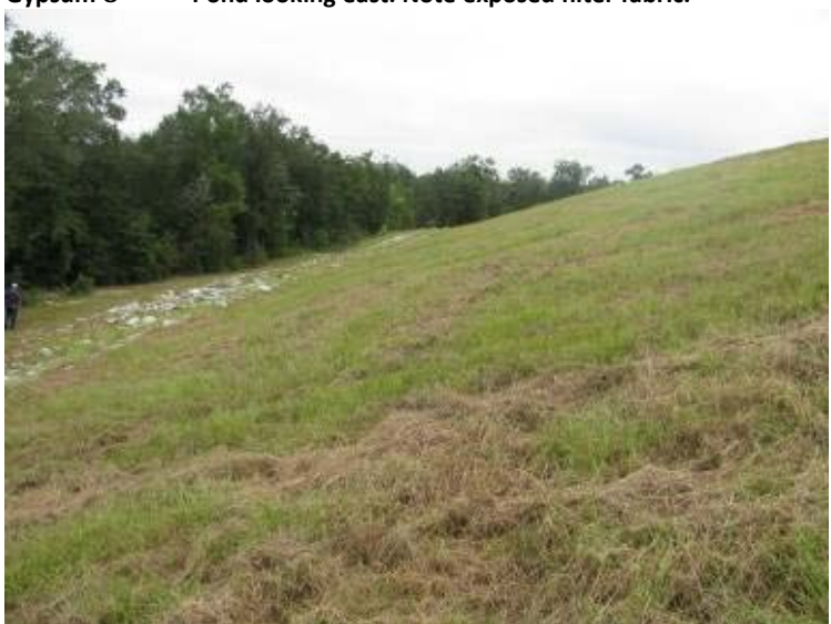
Photo 127: Exterior slope along west side of Gypsum O Pond looking north.
