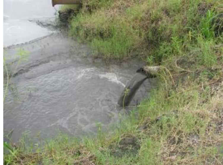
Photo 92: Discharge water from plant operations into Decant/Settling Pond #3.
