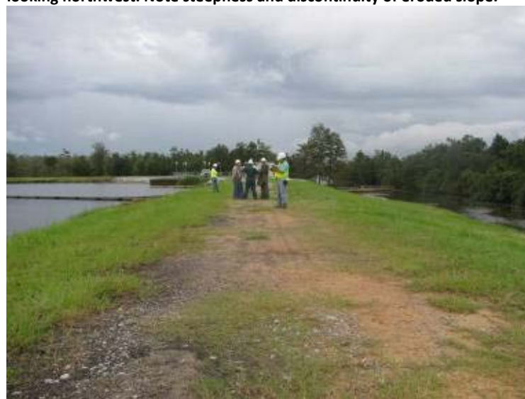
Photo 56: Crest of Ash Pond along southwest embankment looking southeast.
