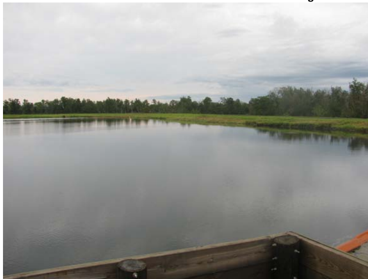
Photo 35: View of Ash Pond from spillway structure looking north.
