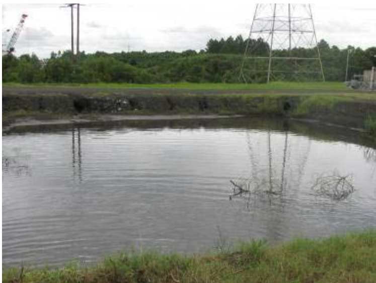
Photo 101: Surface of Decant/Settling Pond #4 looking north.
