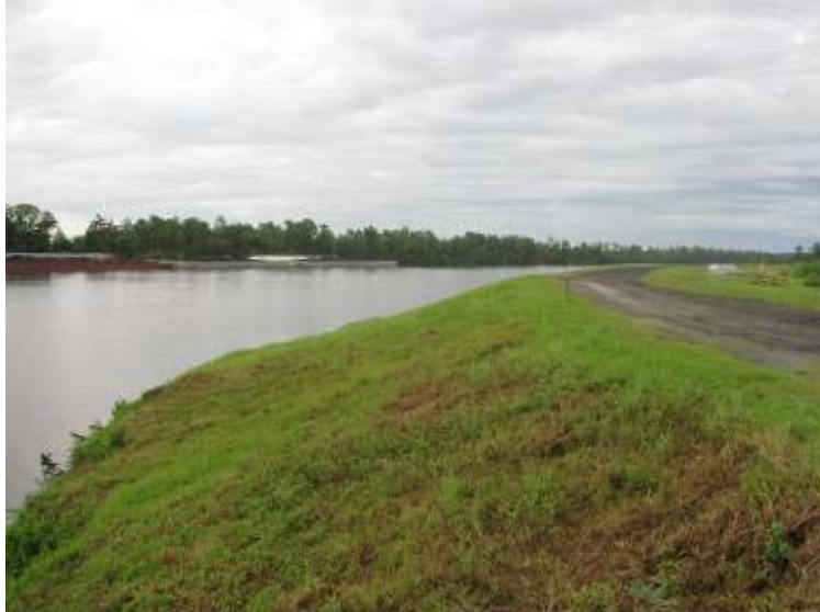
Photo 3: Exterior slope and crest of north embankment of Ash Pond showing minor scarp at toe of slope looking east.
