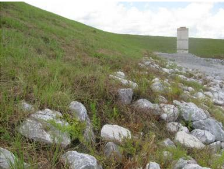
Photo 155: Wet area at toe of slope along east exterior slope of Gypsum Storage Pond looking northwest.
