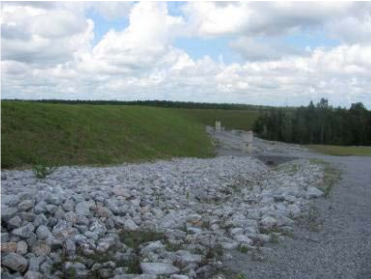
Photo 153: East exterior slope of Gypsum Storage Pond looking northwest.
