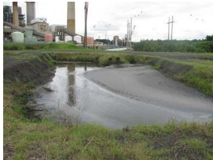
Photo 100: Surface of Decant/Settling Pond #3 looking northwest.
