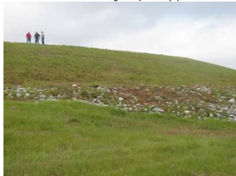
Photo 140: Northeast exterior slope of Process Sedimentation Pond looking south.
