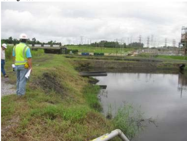
Photo 79: Crest and southeast interior slope of Decant/Settling Pond #5.
