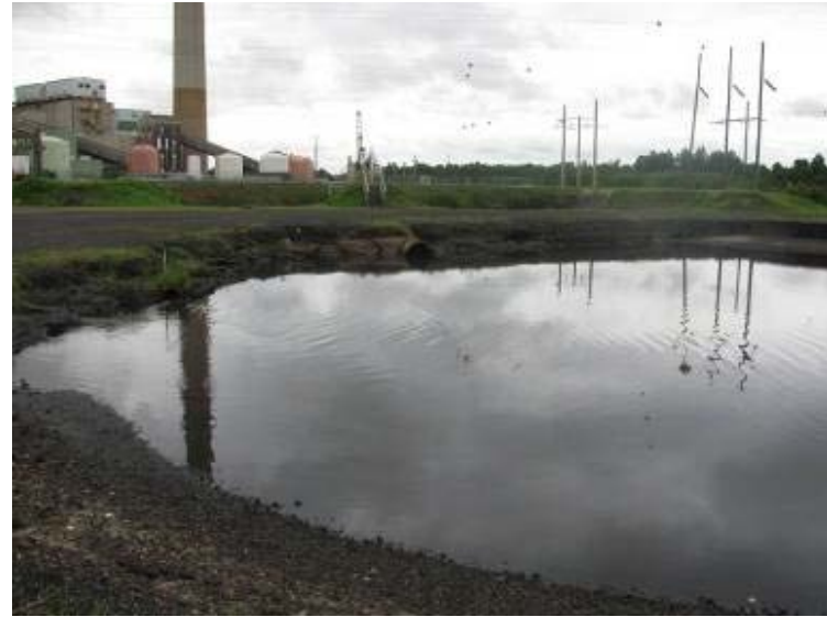
Photo 86: Interior slopes and surface of Decant/Settling Pond #1 looking north.
