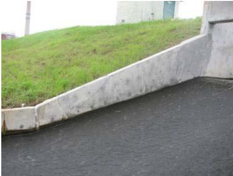
Photo 33: Downstream side and west wall of Ash Pond looking north.
