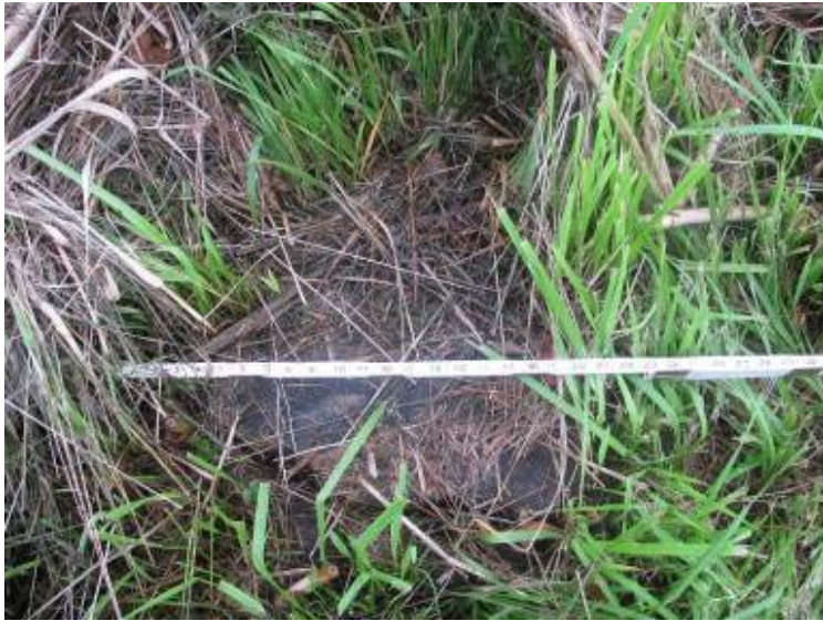
Photo 21: Tree stump found on exterior slope of Ash Pond.
