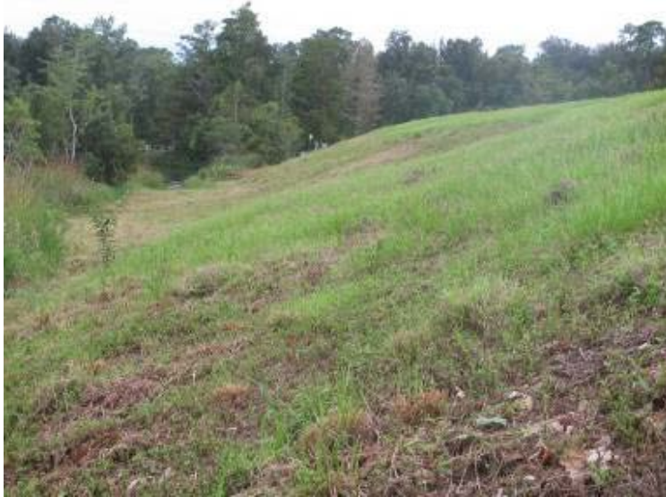
Photo 25: Southeast embankment exterior slope looking southwest.
