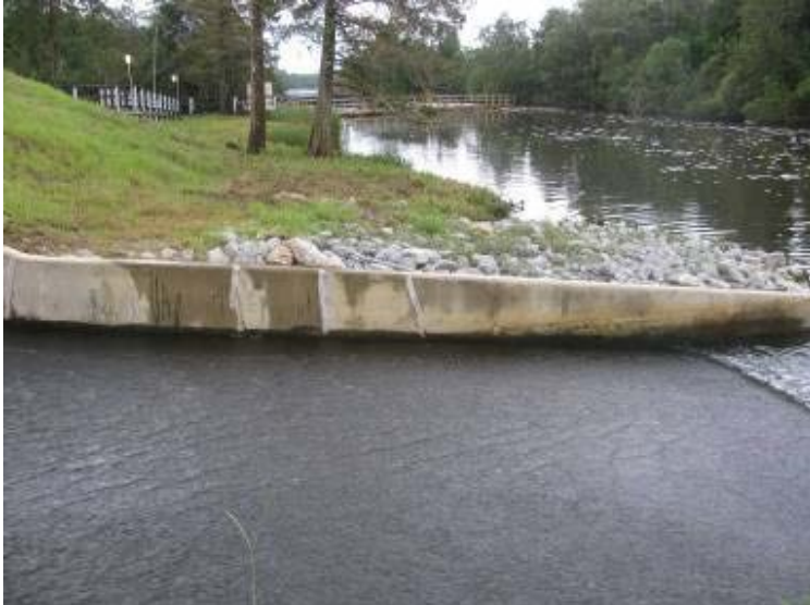
Photo 43: East wall of Ash Pond spillway channel.
