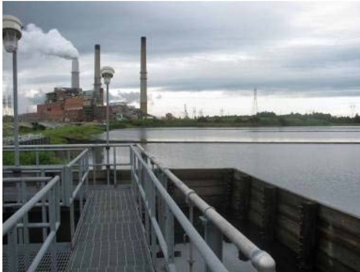
Photo 37: Walkway on upstream side of spillway structure looking northwest.
