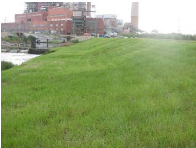
Photo 47: Exterior embankment slope of Ash Pond along southwest embankment.
