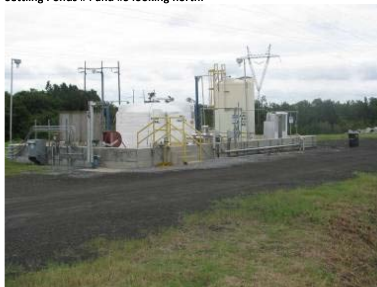
Photo 96: Chemical storage area located near north corner of Ash Pond.
