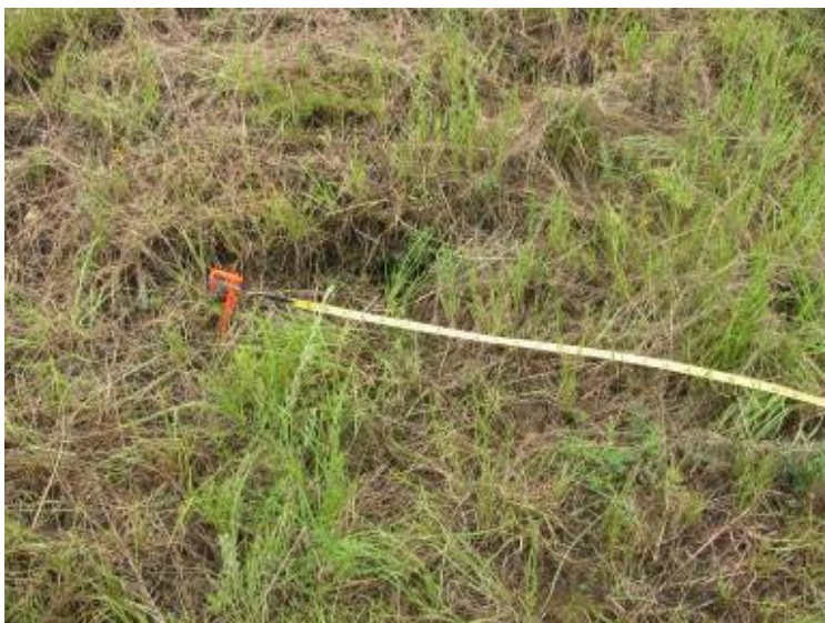
Photo 129: Animal burrow located at approximate mid-face of west exterior slope of Gypsum Pond.
