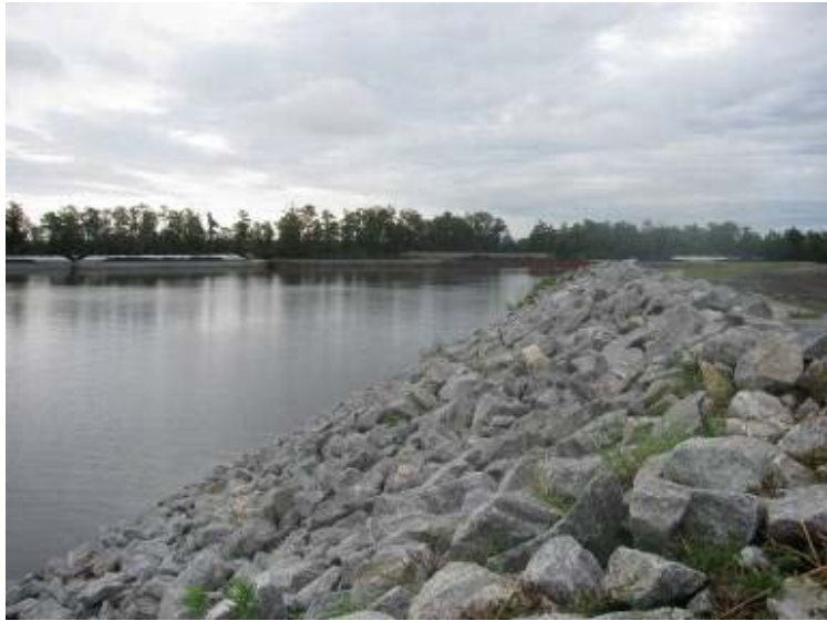
Photo 1: Ash Pond – (typical) riprap along exterior slope of north embankment adjacent to Escambia River looking east.
