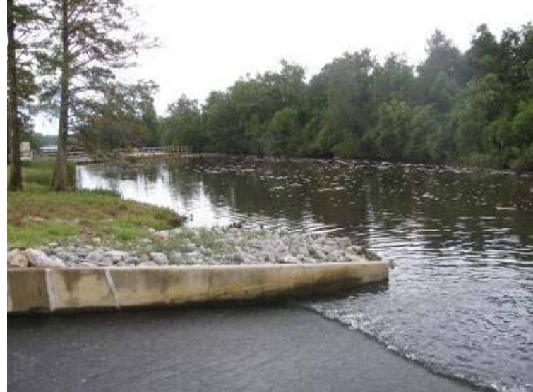
Photo 44: East wall of Ash Pond spillway channel.
