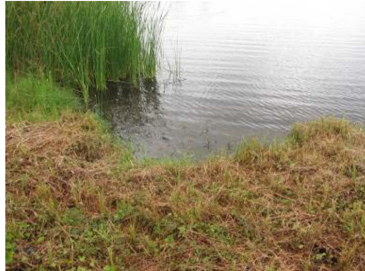
Photo 50: Interior slope of Ash Pond looking north.
