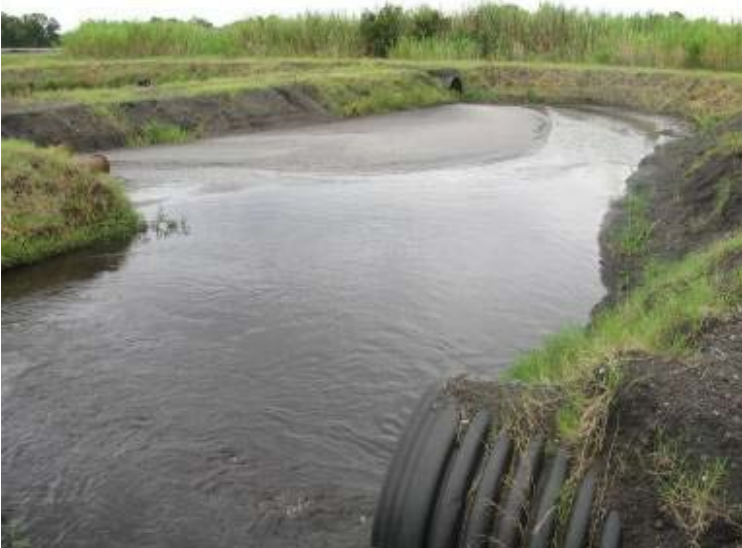
Photo 91: Interior slopes and surface of Decant/Settling Pond #3 looking southeast.
