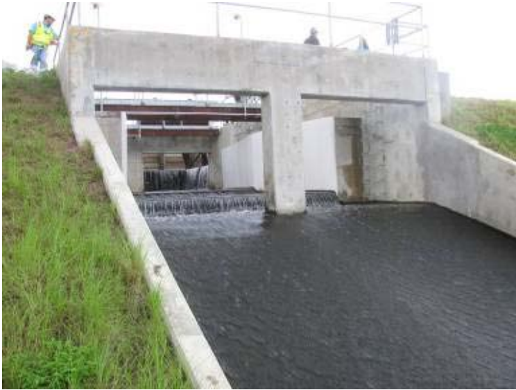
Photo 41: Downstream side of Ash Pond spillway.
