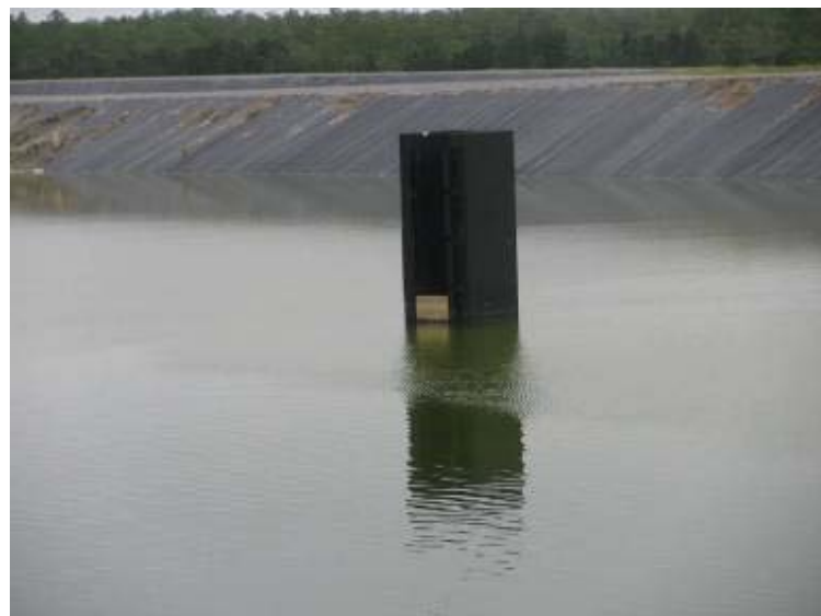
Photo 106: Surface of Gypsum Pond and Decant Riser looking north.
