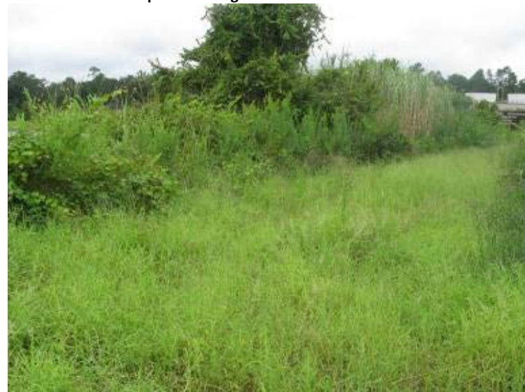
Photo 84: Crest of Ash Pond along northwest side. Note dense vegetation.
