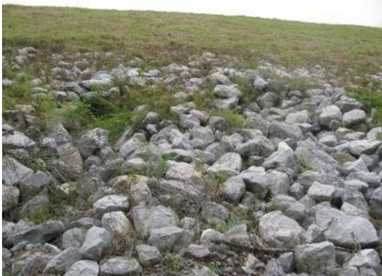
Photo 123: Riprap slope protection along toe of west exterior slope of Gypsum Pond looking east. Note depressed area at center.
