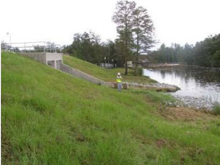
Photo 45: Exterior slope of Ash Pond along southwest embankment.
