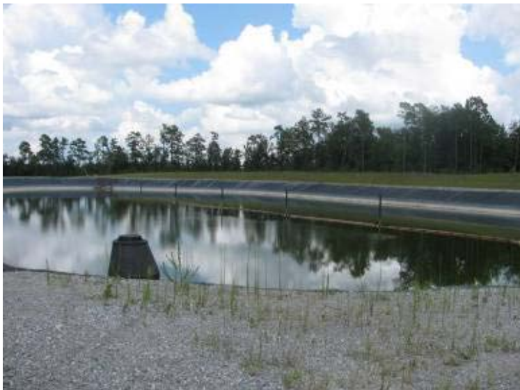
Photo 179: Surface of Process Return Water Pond looking northeast.
