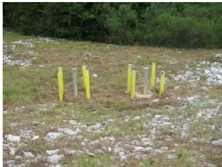
Photo 118: Monitoring Wells located beyond exterior toe of slope on west side of Gypsum Pond.
