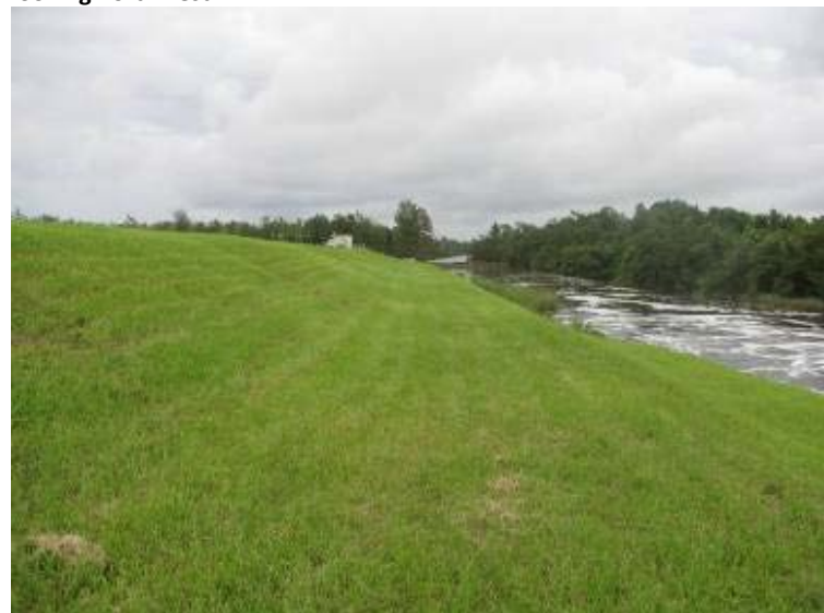
Photo 48: Exterior slope of Ash Pond along southwest embankment looking southeast.
