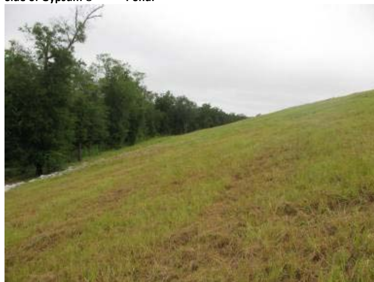
Photo 120: Exterior slope along west side of Gypsum Pond looking north.
