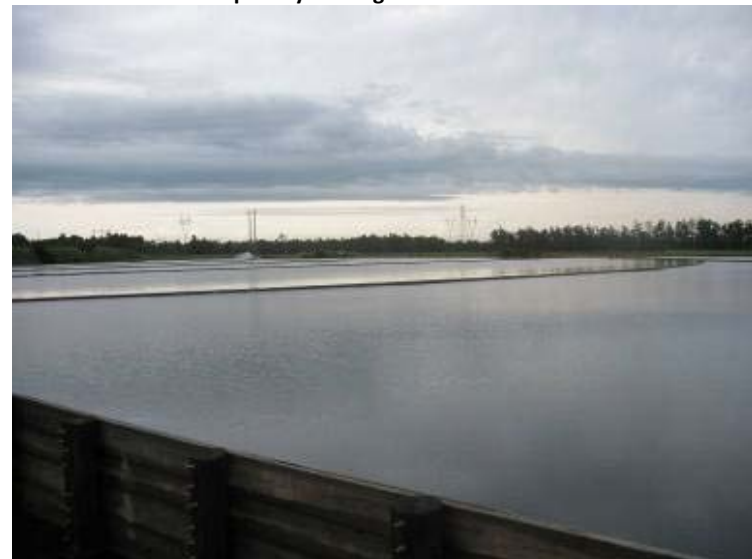
Photo 36: View of Ash Pond spillway structure looking northwest.
