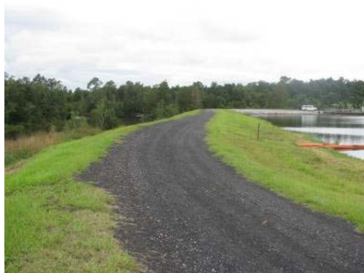
Photo 68: Crest of Ash Pond near east corner of pond looking southwest.
