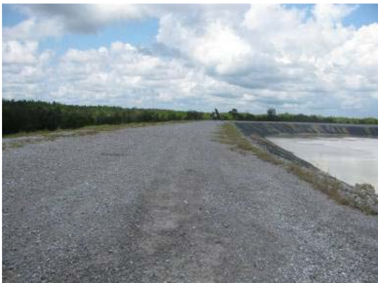
Photo 173: Crest of west embankment of Gypsum Storage Pond looking north.
