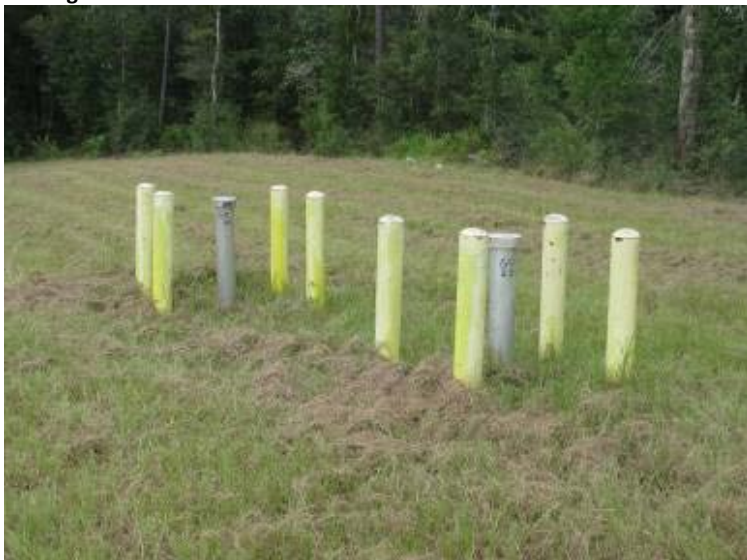
Photo 183: Monitoring well pairs located beyond exterior toe of slope of Process Return Water Pond looking north.
