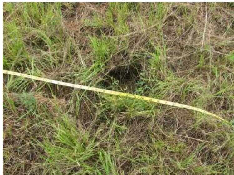
Photo 130: Animal burrow on west exterior slope of Gypsum Pond.
