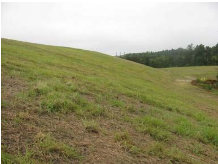
Photo 119: Exterior slope along west side of Gypsum Pond looking south.
