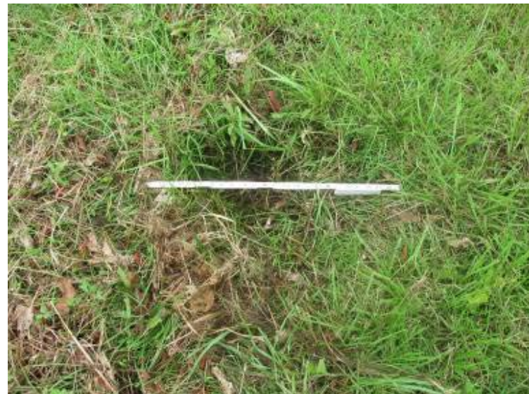
Photo 52: Animal burrow located on crest of Ash Pond.
