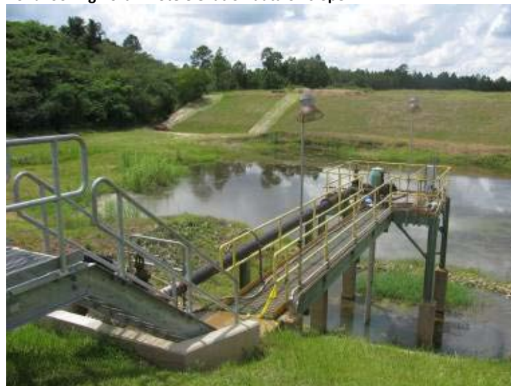
Photo 196: General view of fly Ash Landfill stormwater pond area looking west.
