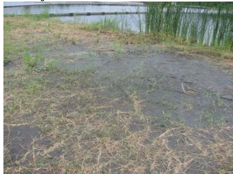
Photo 72: Ash delta located along interior slope of northeast embankment of Ash Pond looking south.
