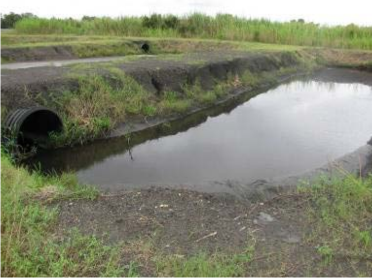
Photo 89: Interior slopes, divider and surface of Decant/Settling Pond #3 looking east.
