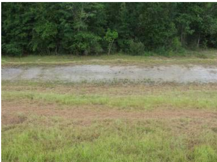
Photo 109: Perimeter road/maintenance bench at toe of southwest slope of Gypsum O Pond looking southwest. Note standing water at toe.
