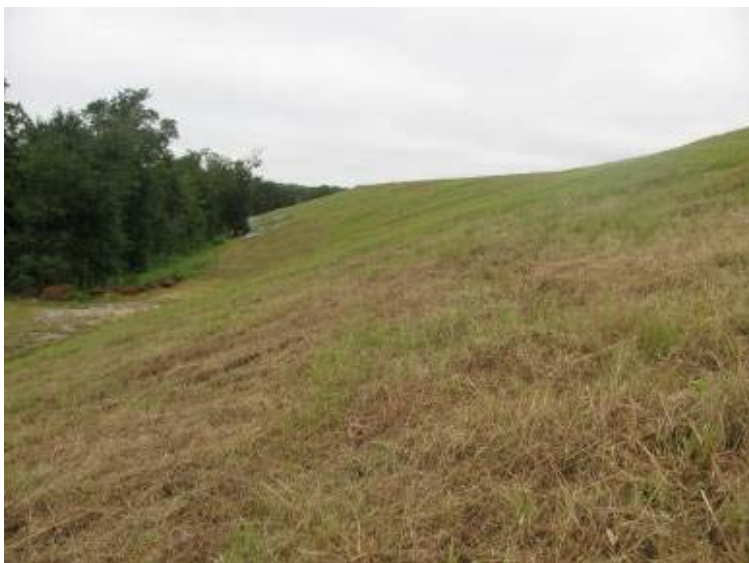
Photo 117: Exterior slope along west side of Gypsum Pond looking north.
