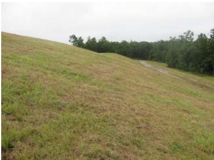
Photo 113: Exterior slope along southwest side of Gypsum Pond looking southwest.
