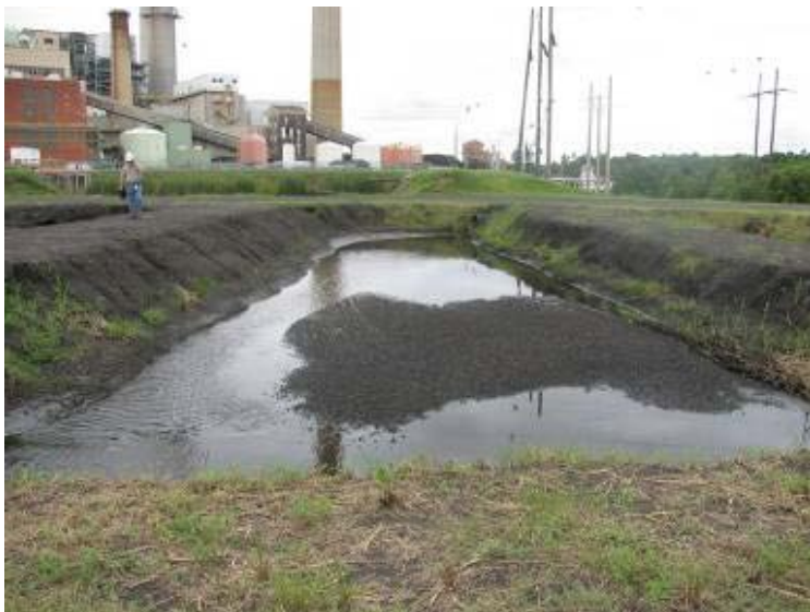
Photo 99: Surface of Decant/Settling Pond #2 looking northwest.
