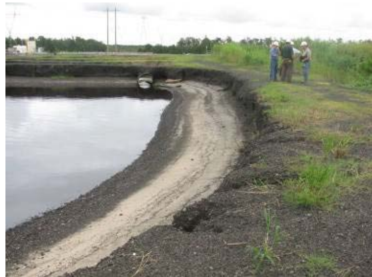
Photo 88: Interior slopes and surface of Decant/Settling Pond #1 looking northeast.
