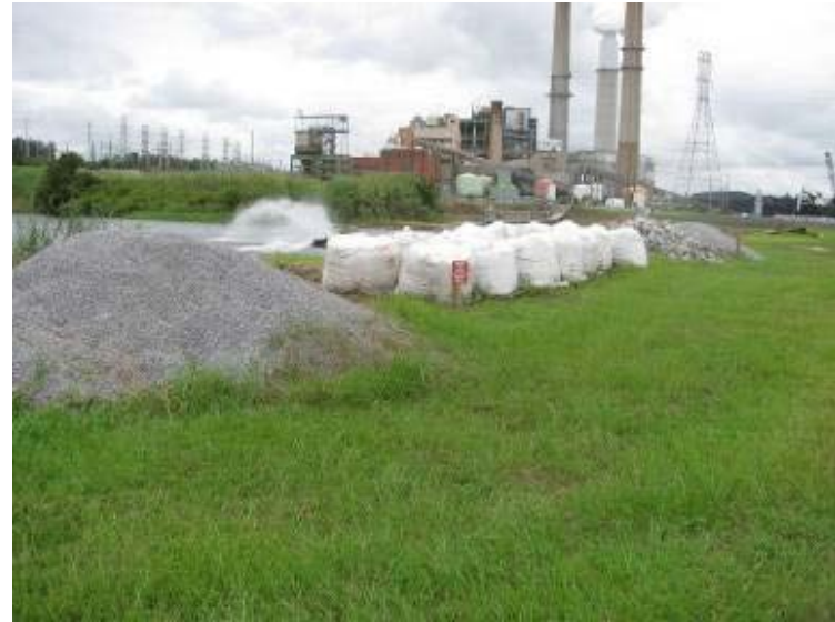
Photo 74: Emergency response materials (gravel, sand, riprap) located near north corner of Ash Pond.
