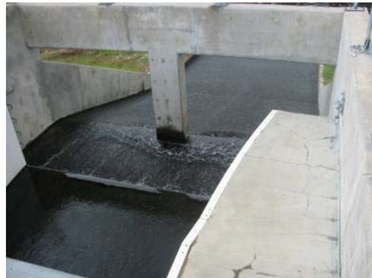
Photo 40: Spillway structure looking downstream.
