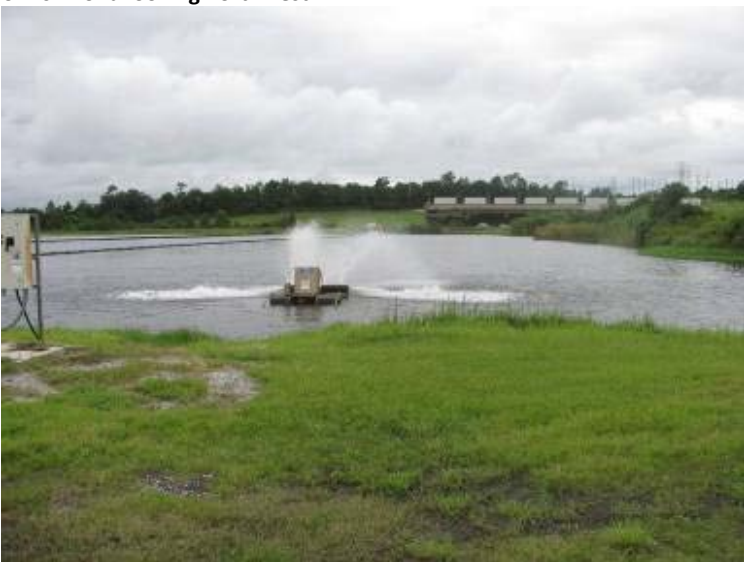
Photo 75: Aerator/oxygenator located near north corner of Ash Pond.
