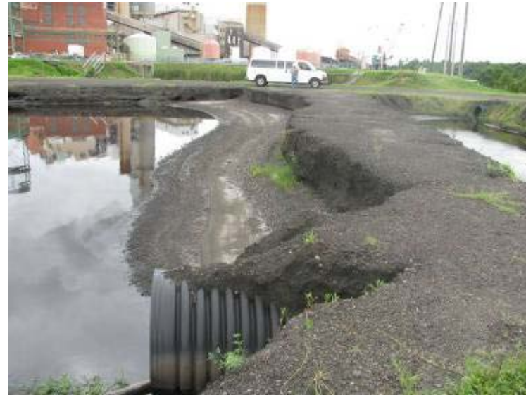
Photo 98: Divider dike between Decant/Settling Ponds #1 and #2 looking northwest.
